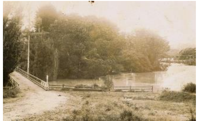
Accession 2958/5/2: Edwardian postcard - the old Karapiro bridge (left), with earlier low level bridge to Leamington in the distance (right). The Karapiro Stream runs left to right. Look how high the water level is!
