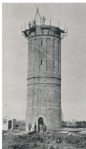
Building the Water Tower 1903, CM2958.38
